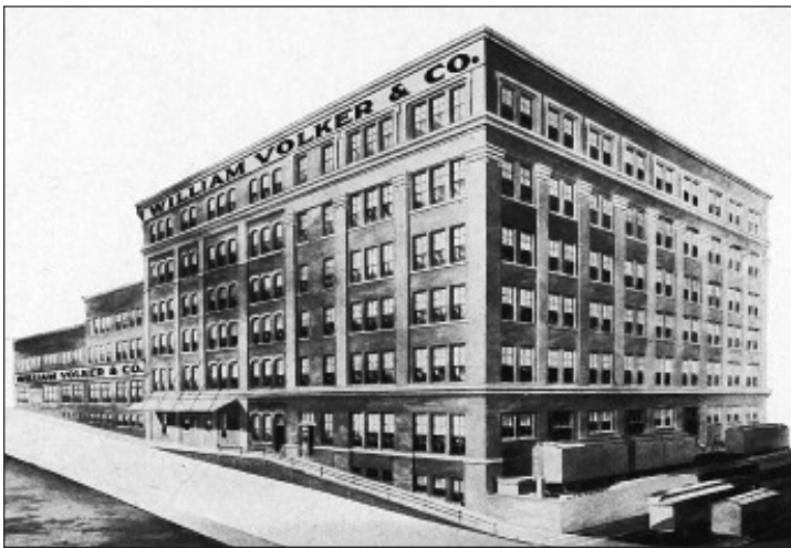
This building at Main and Second in Kansas City served as William Volker and Co. headquarters from 1915 to 1951. [SHSMO-KC]
