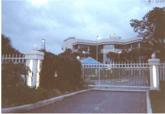
Figure 2. Headquarters of the Seminole Tribe of Florida, Inc.
